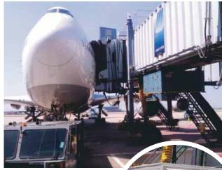
AOT installed Fixed Ground Power Units and Fixed Pre-Conditioned Air units (PC AIR) for 51 parking bays at Suvarnabhumi Airport to provide power supply and cooling for aircraft. This technology enables AOT to reduce air polluting emission and extend the life of aircraft equipment by eliminating the need to keep engines running. AOT is planning to install additional units at all parking bays at Suvarnabhumi Airport and other airports in the future.
